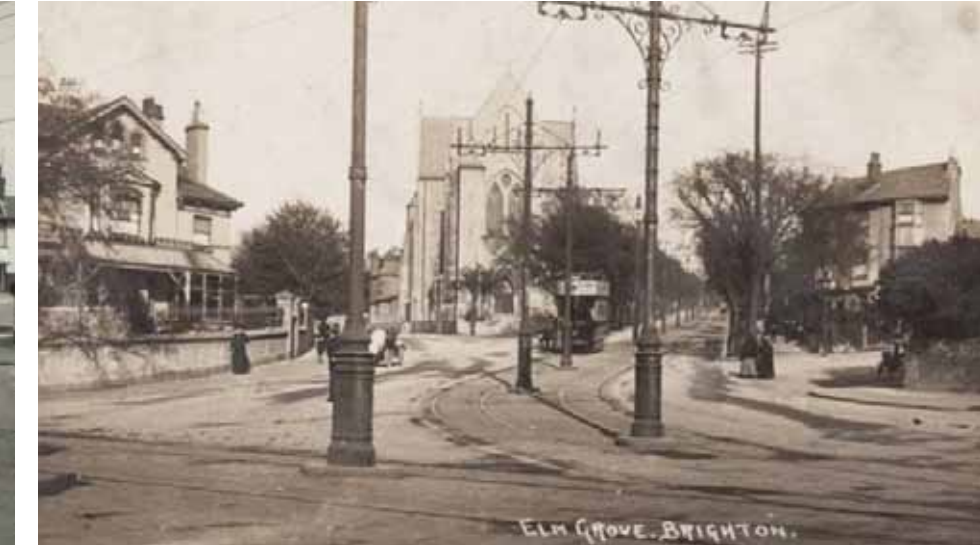
Photo looking up Elm Grove showing the trams
